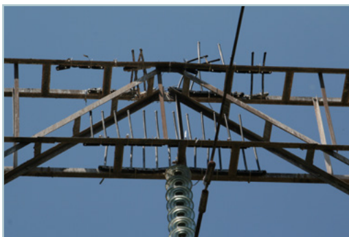
Figure 1: The bird guards supplied by Mission Technologies were not able to withstand the impact of large vultures. Photo credit: the EWT
