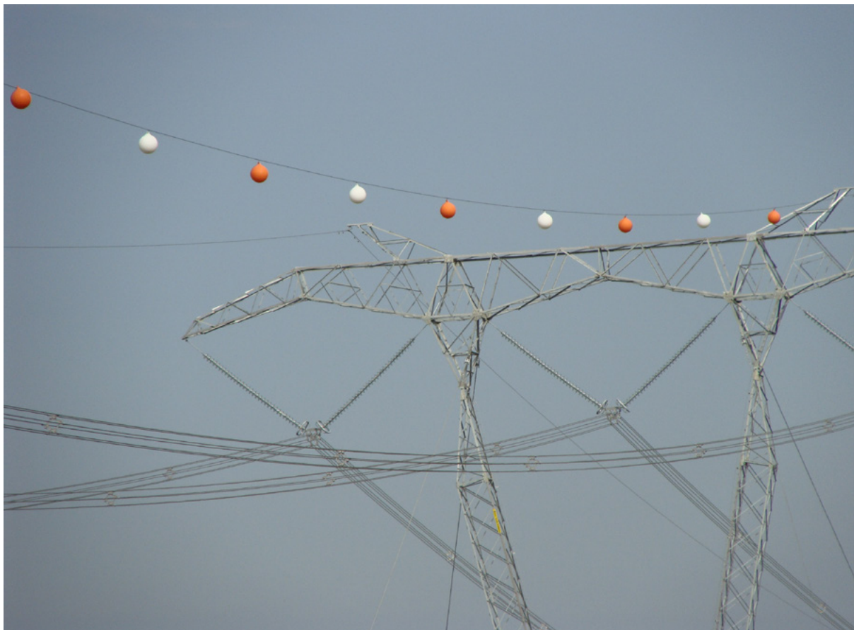
Aviation balls are fitted to power lines to make the line more visible for aircraft but are also effective in preventing bird collisions. Photo credit: Marianne Golding
