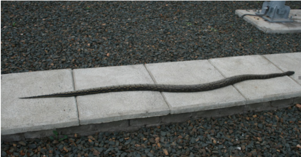
African Rock Python electrocuted in a substation. Photo credit: Eskom
