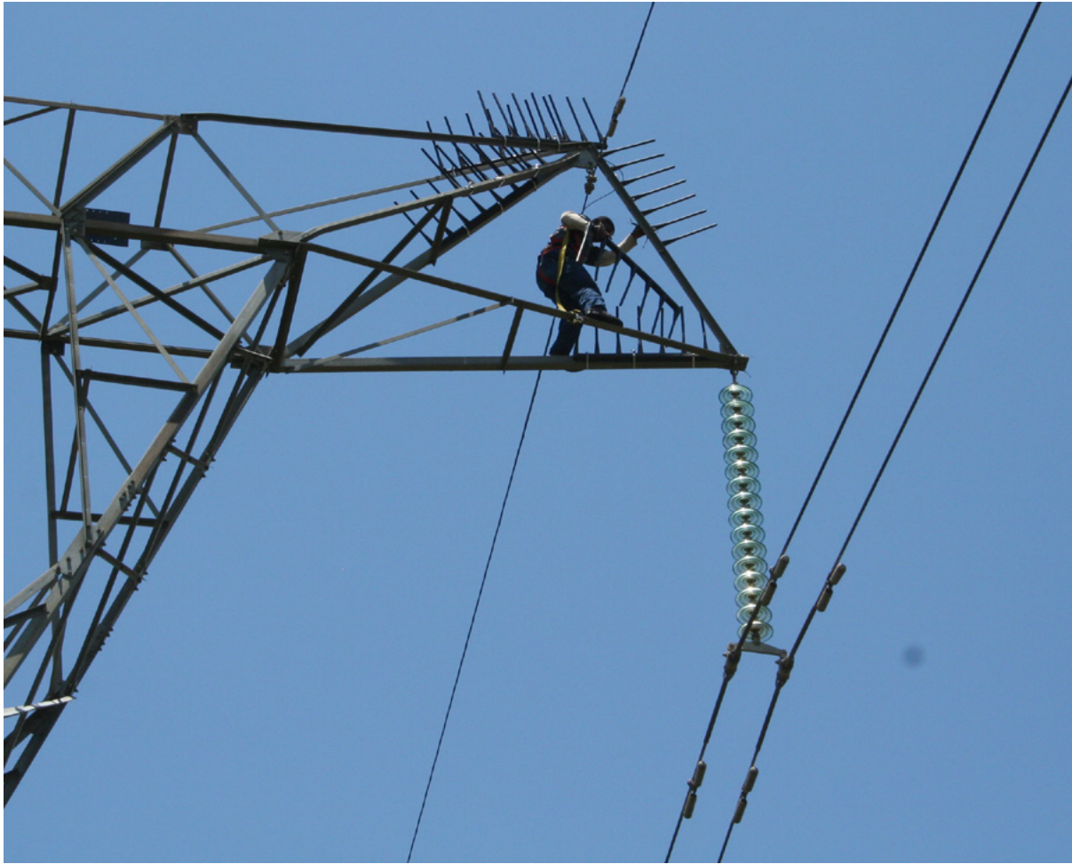
Bird guards fitted to a transmission tower by a live line team. Photo credit: Constant Hoogstad
