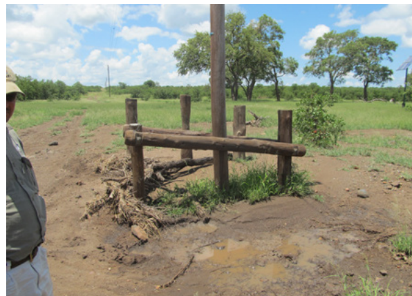
A kraal being built around a wood distribution pole to protect this pole in a high impact area.
