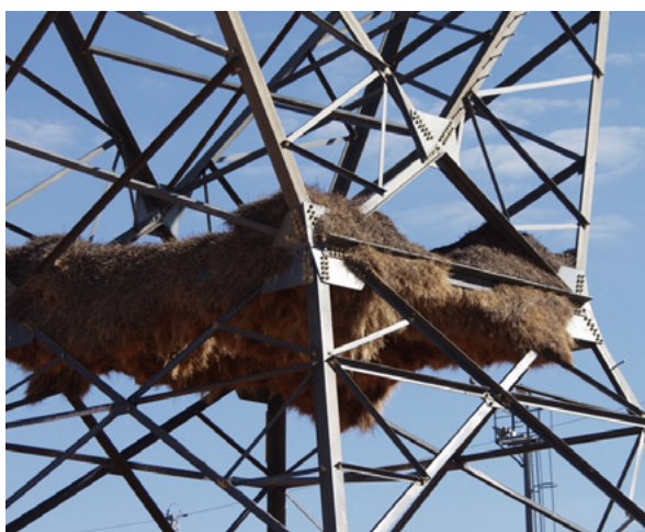
Sociable weaver nest on mast of a transmission tower. Photo credit: John Smallie
