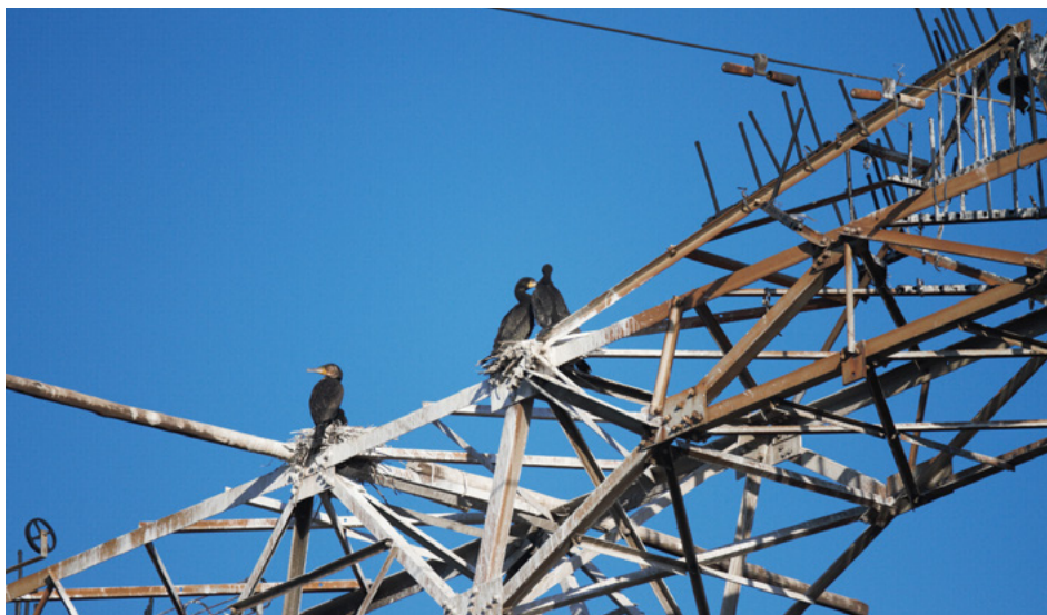
Reed Cormorant nesting on a transmission tower, causing pollution and streamer problems. Photo credit: Matt Pretorius
