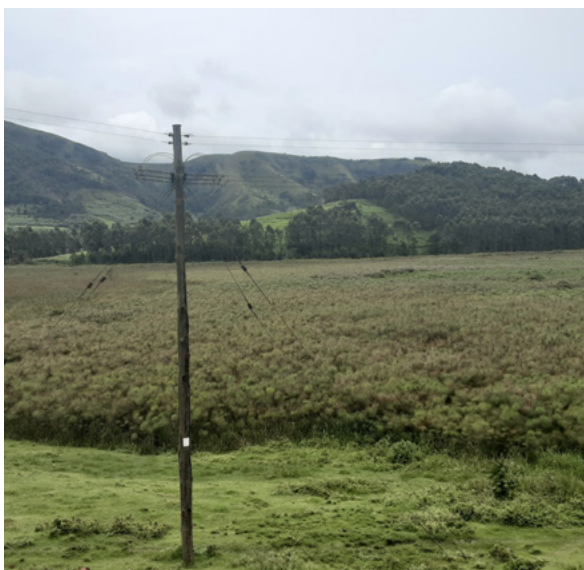
Power line through a wetland Photo credit: The EWT
