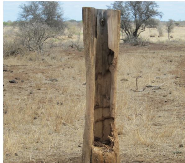
Wood distribution pole destroyed by termites. This is due to the removal of the outer protective layer of creosote as a result of large mammals repeatedly using the pole as a rubbing post. Photo credit: Constant Hoogstad
